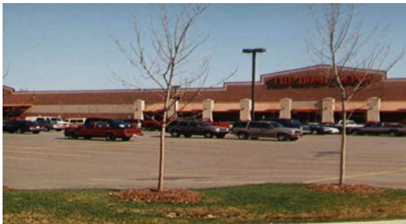
A. New commercial development constructed with onsite storm water detention Upper Rouge River Subwatershed, Northville Township
