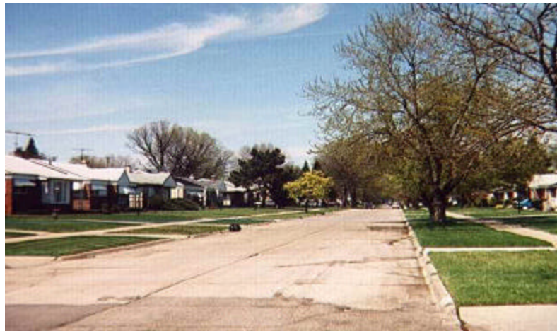
B. Typical residential subdivision built in the 1950s Upper Rouge River Subwatershed, Redford Township
