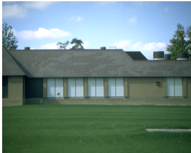
C. Redford Township CSO retention and treatment facility Upper Rouge River—completed and operational (1999)
